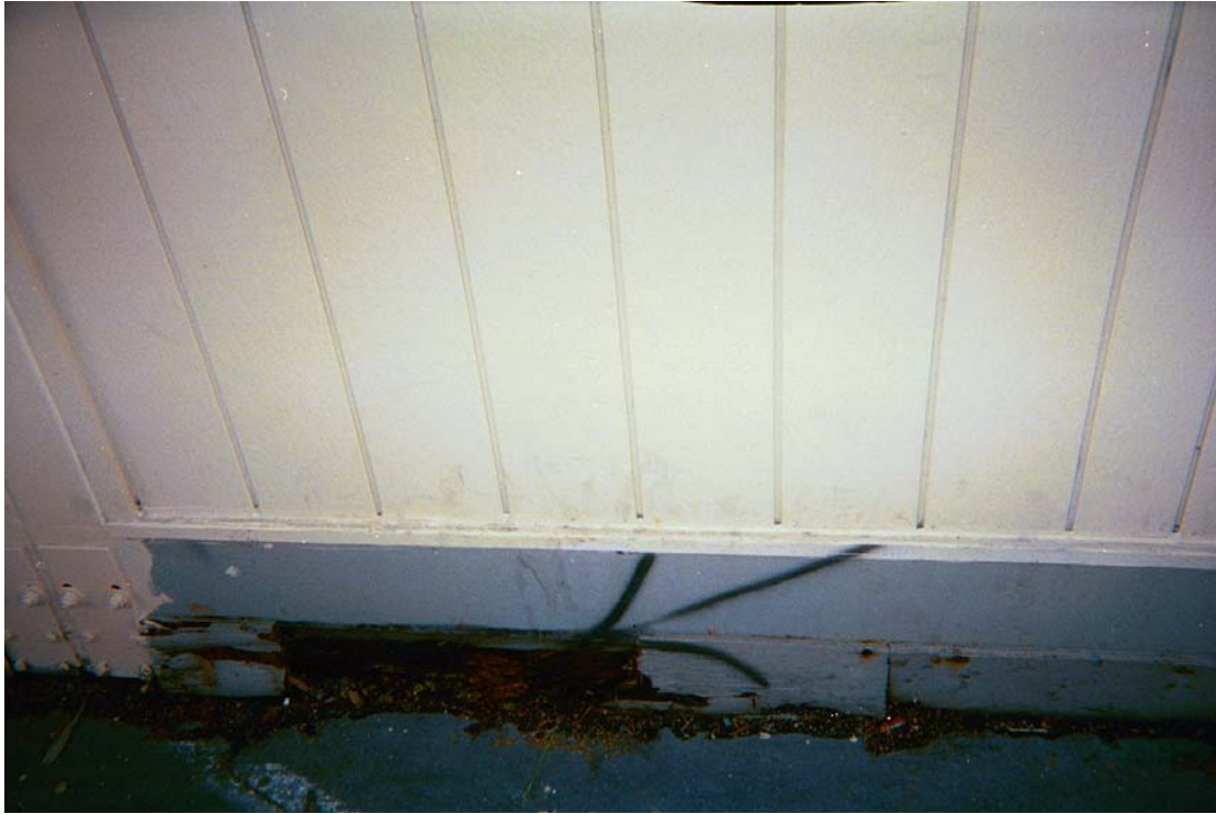
Figure 10: Decay at Base of Portable Building.
