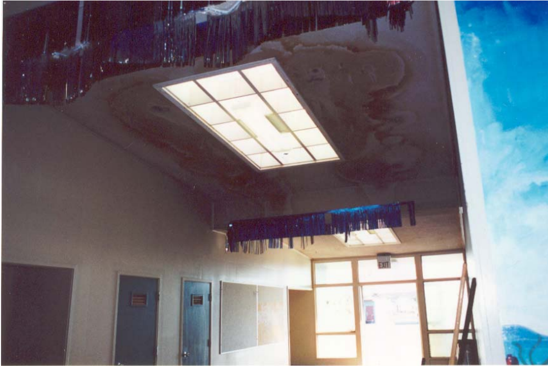
Figure 8: Water Damage at Skylight Over Classroom Corridor.
