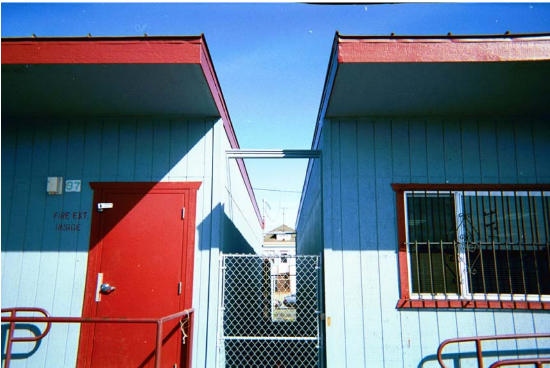
Figure 9: Conduits Between Portable Buildings.
